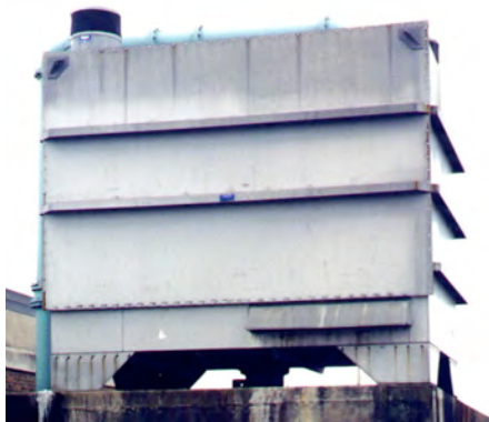
Newly Replaced Aerator at Morton, IL
