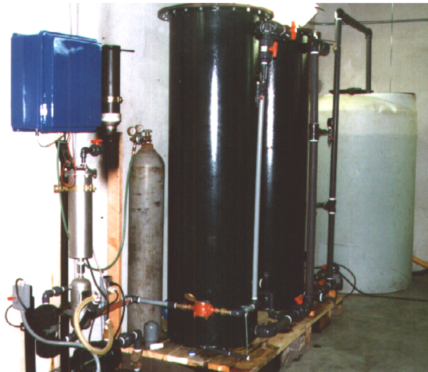
Oxygen Cylinder and Ozonator Generator, Pump, Injector and Contactor (lower left, black), SS Degassing Separator, Ozone Destruct Column (black), Filter Columns in Series (center), Clear Well (right)
