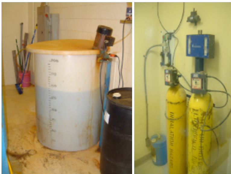
Ferric Chloride and Sulfur Dioxide Feed Systems
