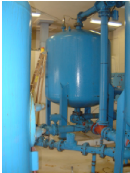
Two carbon steel,vertical filter vessels containing Filtronic's Electromedia 1
