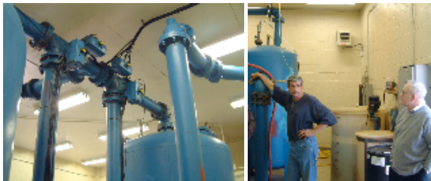
Filtronics' system provides for ferric chloride, chlorine, and sulfur dioxide feeds
