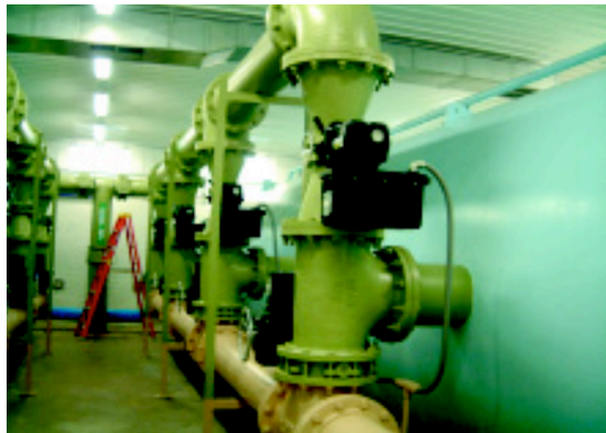
Horizontal pressure filters are divided into four compartments containing dual, crushed anthracite coal and coarse sand, media
