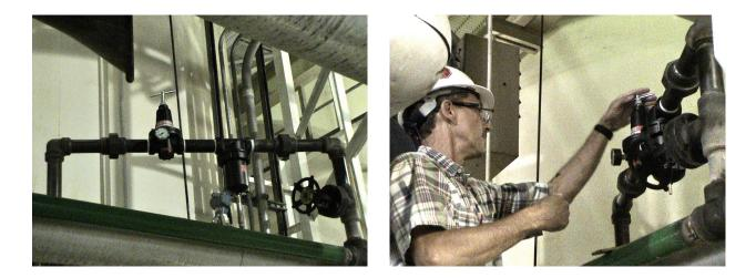
A vertical pipe containing both a solenoid control valve and a manual valve allows the compressed air to enter the false bottom of each filter unit. The existing backwash water diffusers in the filter units were initially designed to accommodate and distribute air.
